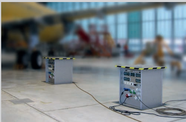
Hangar SE100 Pit
